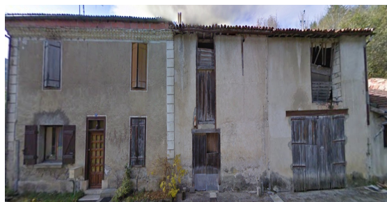
Figure 15 - Source Google Street View
