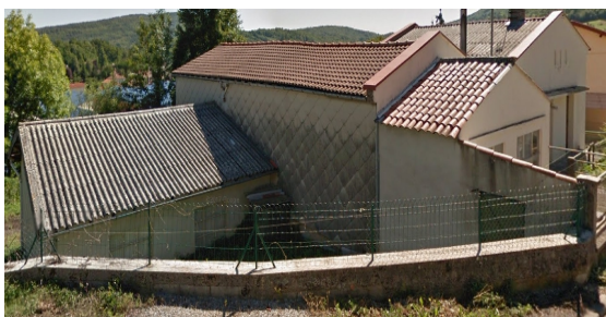
Figure 14 - Source Google Street View
