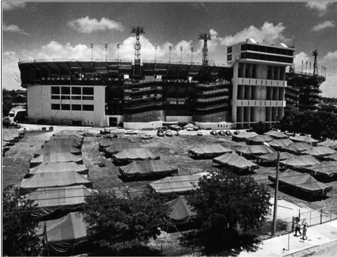
Figure 34. Photo: Orange Bowl Stadium, converted into a temporary processing centre during the Mariel boatlift.
