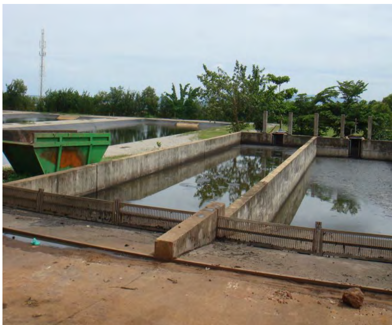
Photo 20: Station d'épuration de Sonfonia
