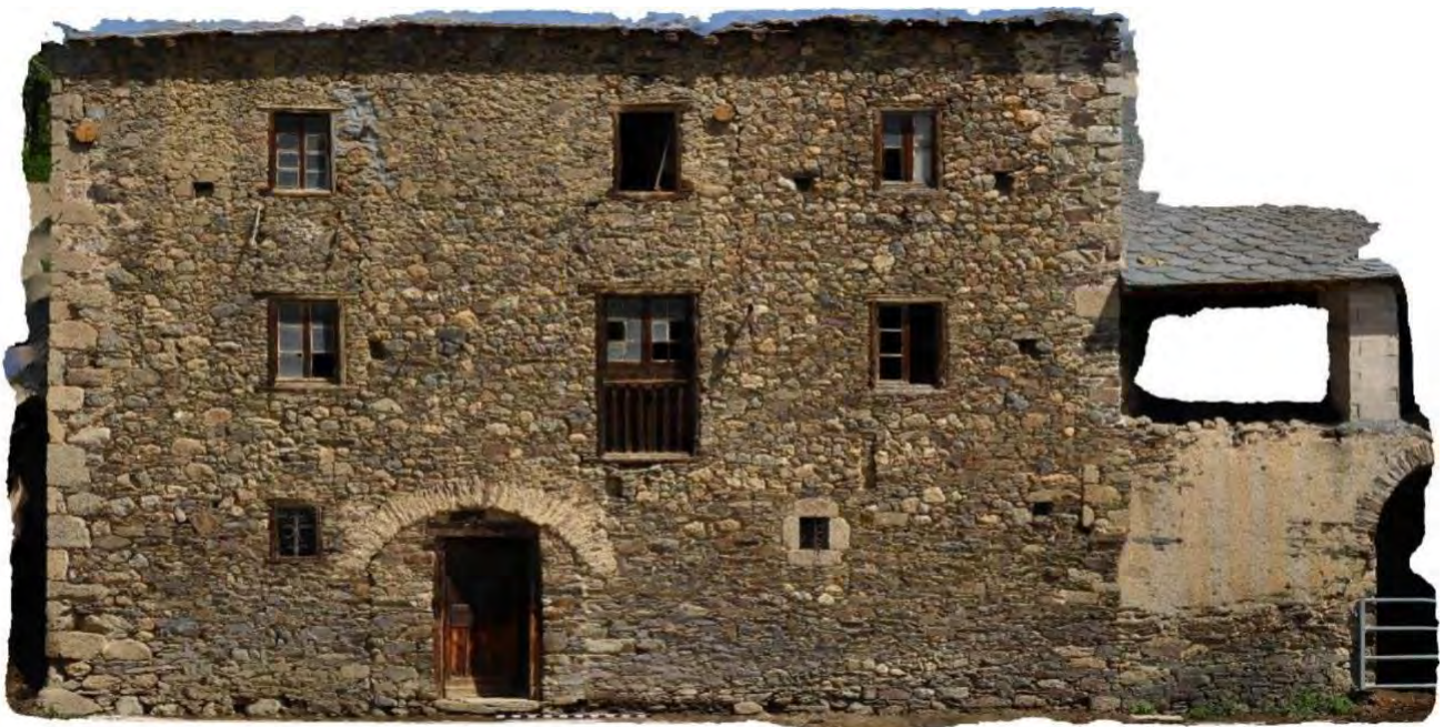
Figure 48: Southern façade of the Building CF3 within the southern complex. Photos: Bizzarri, 2022. Photogrammetric elaboration: Bizzarri, 2022.
