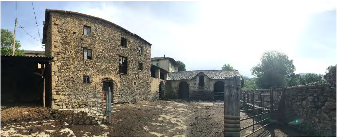
Figure 46: Southern complex of Mas Rondole, seen from the South-West. Photo: Bizzarri, 2022.
