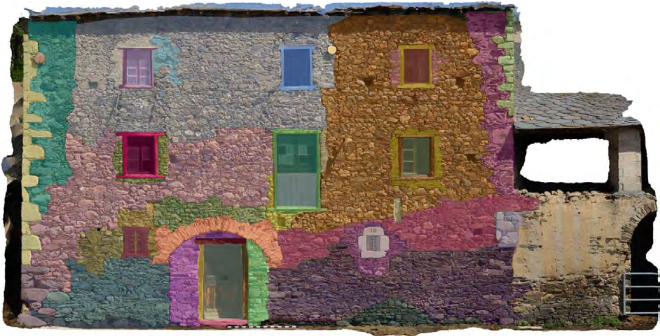
Figure 49: Stratigraphic masonry units identified on the façade. Bizzarri, 2023-24.
