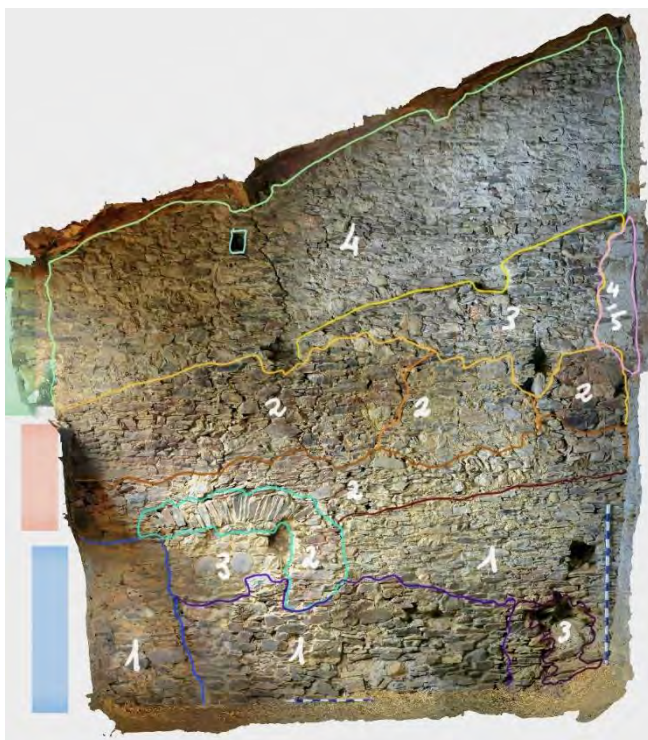
Figure 51: Overview of the inner western façade by the Building CF2 of the Southern Complex. The lower section can be seen as belonging to a first phase of construction (1- blue), possibly tied to the preceding structure in the area or the connection with Building CF3. The presence of a number of broken and slightly collapsing sections hint at the previous presence of structures attached to the wall that are no longer visible – possibly a manger. Phase 2 (red-yellow) involves the construction of the arched structure in the southern section of the façade, and the masonry units above. The holes present on the higher end of this part of the façade hint at the presence of a roofing structure that used to be placed below the current one. Also, the roofing structure seems to have followed a two-slopes rather than being the one-slope roof visible today. Phase 3 (yellow-green) is connected to the modification of the masonry structure right above the second phase and possibly the dismantling of the structure connected to the arch placed below, with its filling through rubble and other fragments and materials. Phase 4 is the highest section of the wall, tied to CF3. Photo: Bizzarri, 2022. Photogrammetric elaboration and notes: Bizzarri, 2023.
