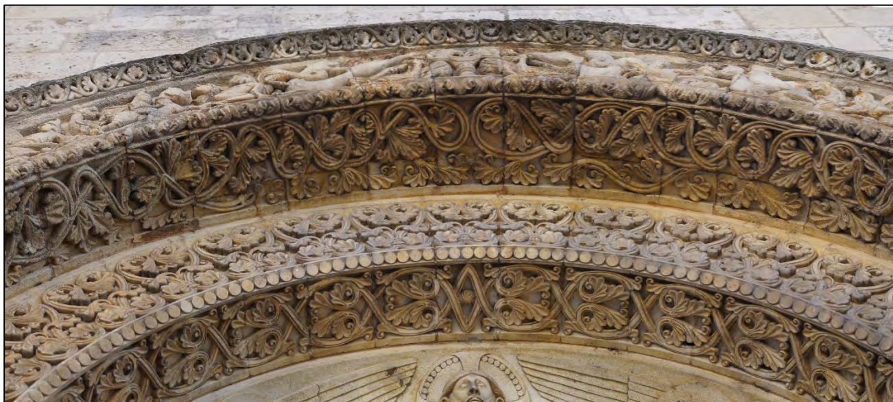
Figure III.1.11 – Ensemble sculpté surmontant le portail, façade occidentale.
