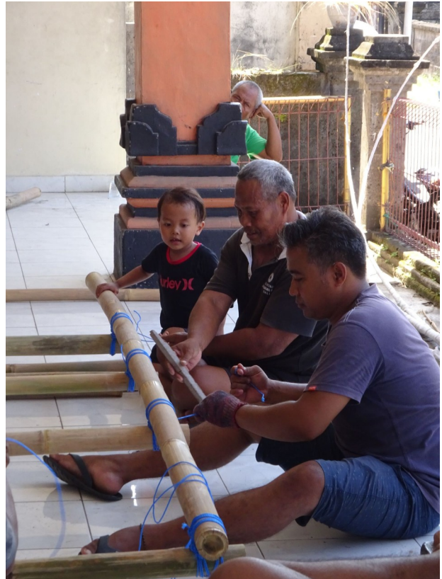
Illustration 141: Construction structure de portage 3 - 18/03/23
