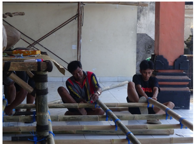
Illustration 139: Construction structure de portage - 18/03/23
