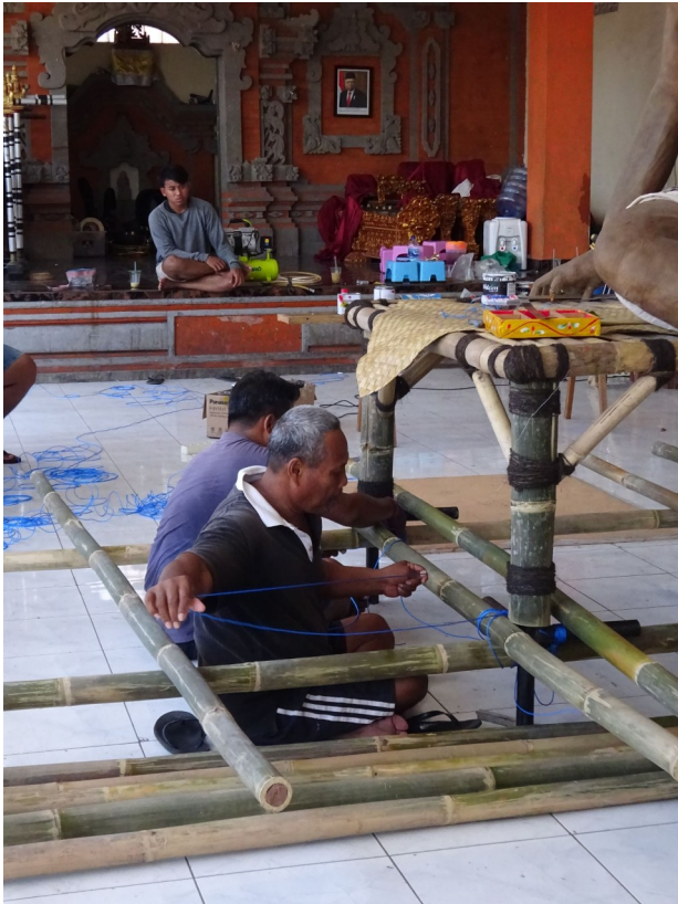
Illustration 140: Construction structure de portage 2 - 18/03/23
