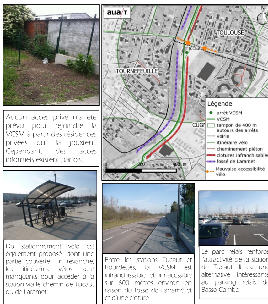
FIGURE 87 : ACCES A LA STATION DE TUCAUT
